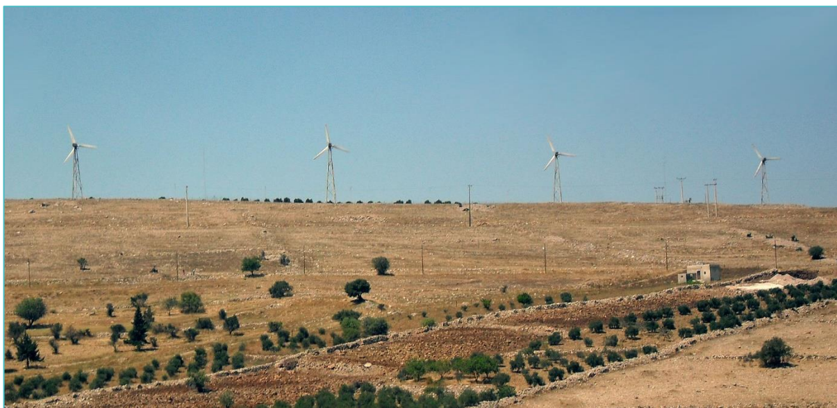
Figure 26: 320 kW Ibrahimyah (Jordan) wind power plant
